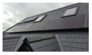
PV Panels do not need Direct sunlight. They can generate electricity from daylight. This means that even on cloudy days, this system will still generate some electricity.
